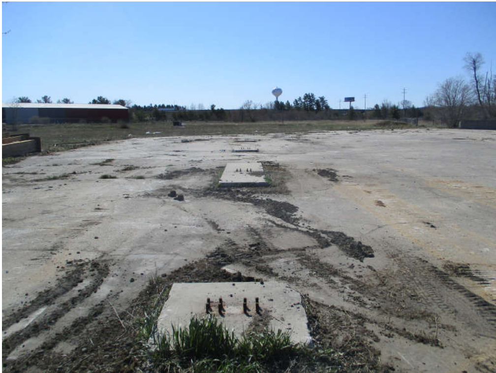
View of existing footers to be removed facing southeast.
