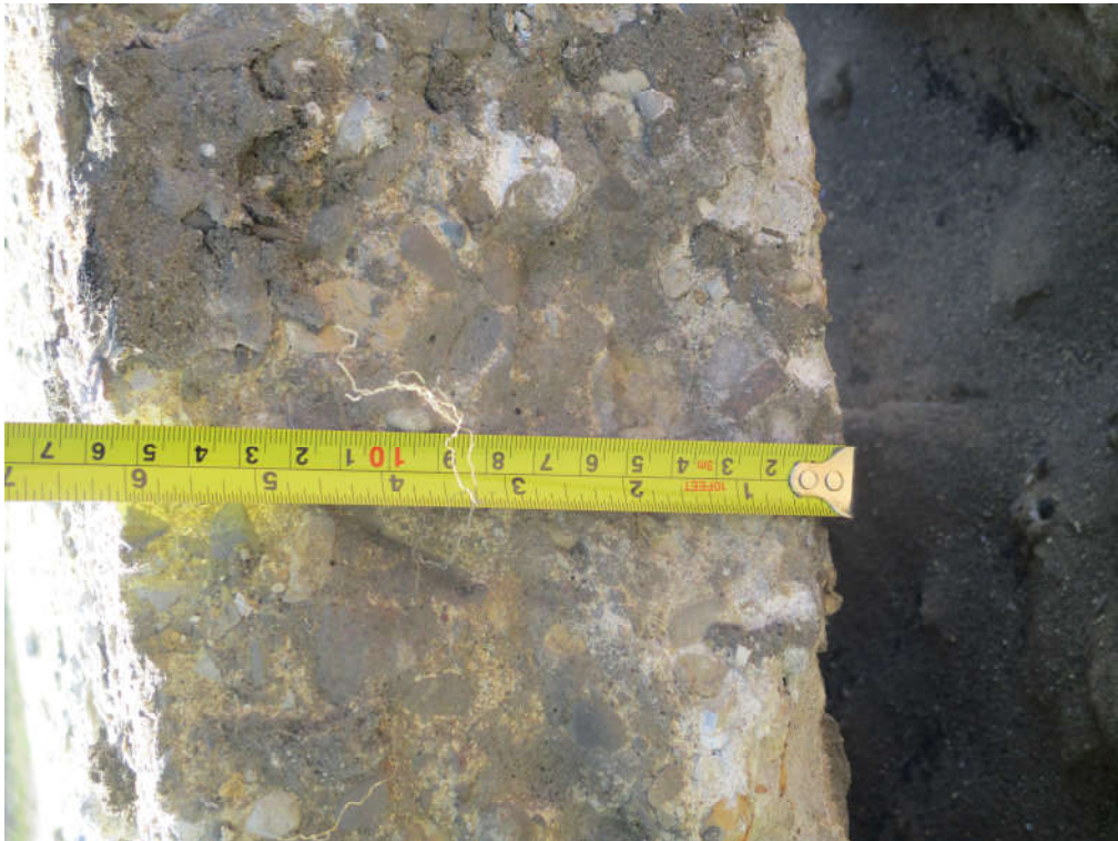
View of existing concrete thickness to be removed.
